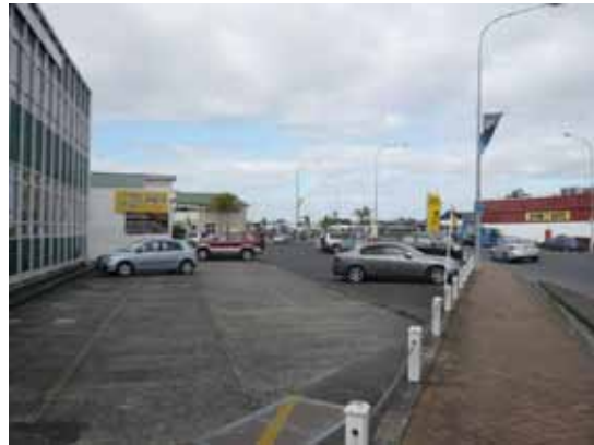
Rear of NRC building
